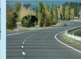
Application in Highway
